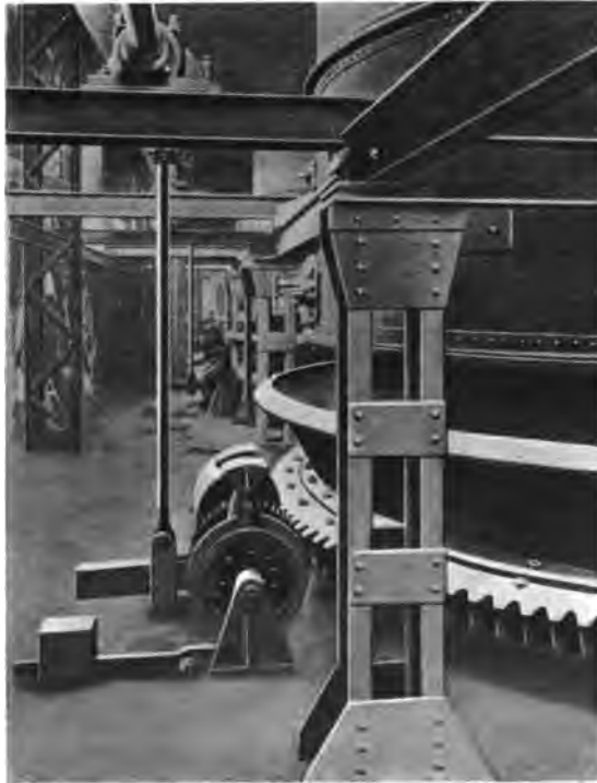
FIG. 51.—“Pilgrim's Step” Mechanism for “Hilger” Gas Producer.
